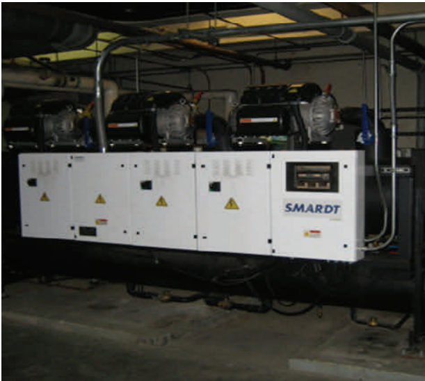
Turbocor Chiller
